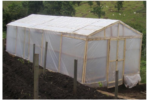
Side view of the greenhouse
