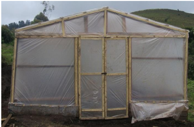
Front view of the greenhouse
